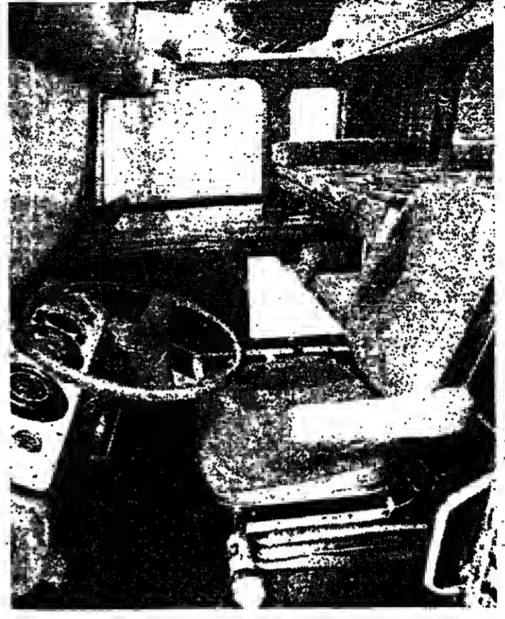
An example of what can be achieved in cab comfort in a Leyland Marathon (left)—this cab was originally completed as part of an exercise for trucks involved in Middle East operations. Right: from arm-choir comfort in Bedford's TM long-haul vehicle, the driver has access, via a sliding panel, to a cold box: The cab has fluorescent lighting at night and privacy is provided by roller blinds and one-way glass
